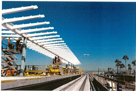
The canopy being installed at the Aviation/Century Station on the Crenshaw/LAX Line. Photo: Metro.
